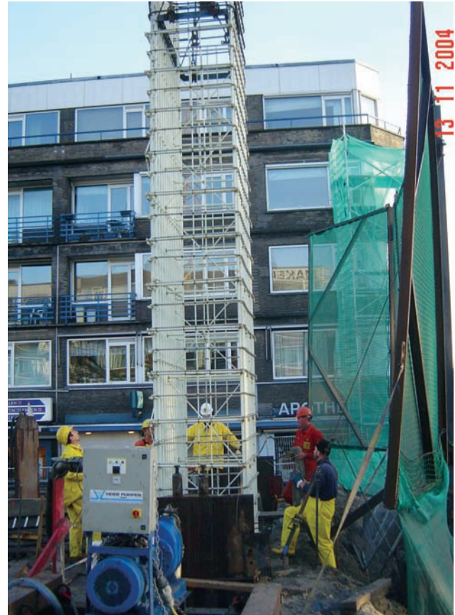
[Fig. 17] Installation of GFRP-Cage
