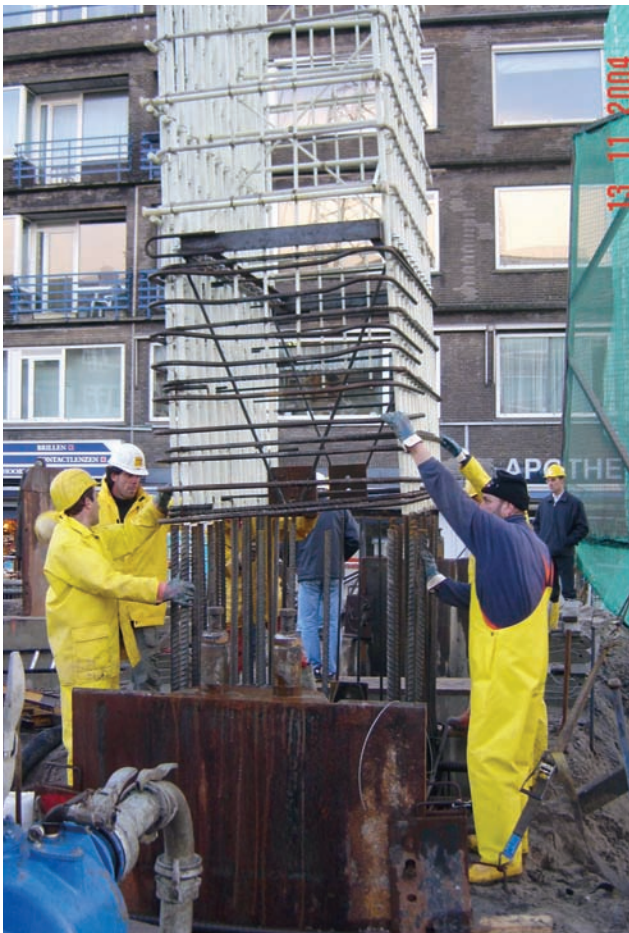
[Fig. 16] Connection GFRP-Cage with Steel Reinforcement Cages
