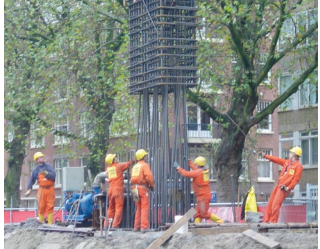
[Fig. 9] Joint of Two Reinforcement Cages for 1.2 m Diaphragm wall
