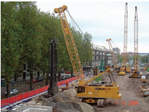
[Fig. 5] Diaphragm Wall Activities at Blijdorp Station
