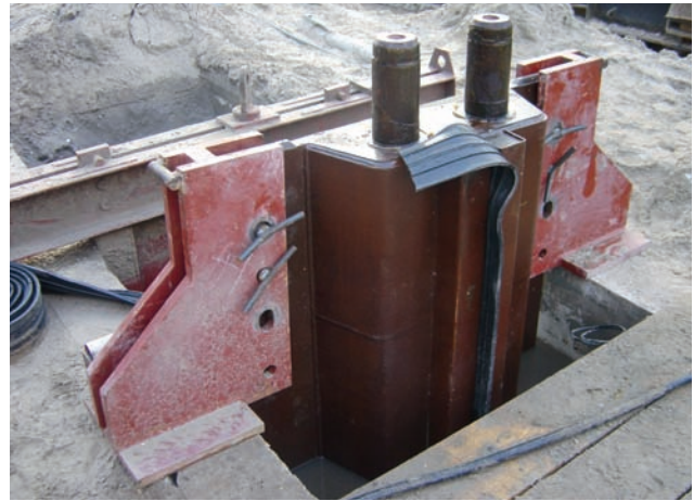
[Fig. 6] Recoverable Steel Joint Element
