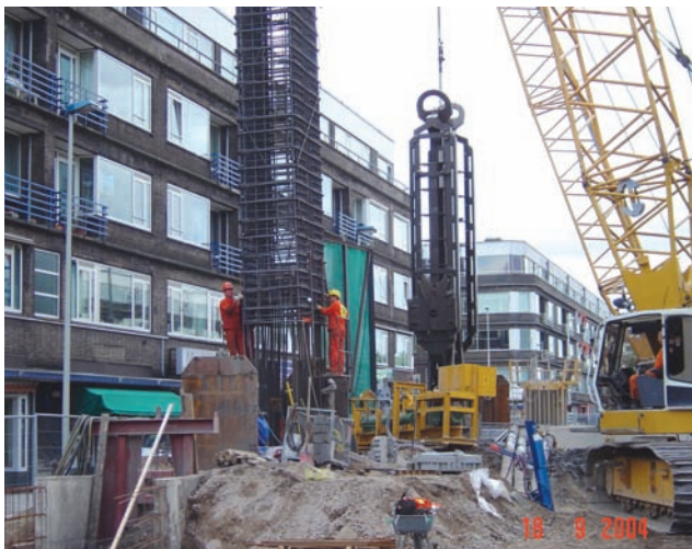
[Fig. 8] Installation of a Reinforcement Cage for a 1.5 m Diaphragm Wall
