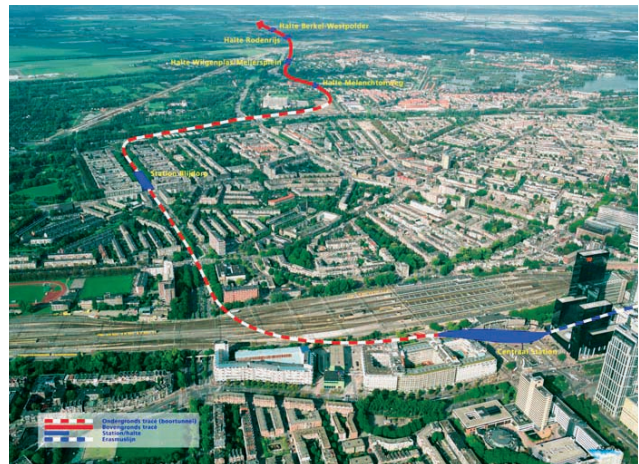
[Fig. 1] Aerial View on Tunnel Track in Rotterdam
