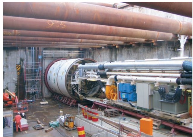
[Fig. 19] TBM in Start Seal
