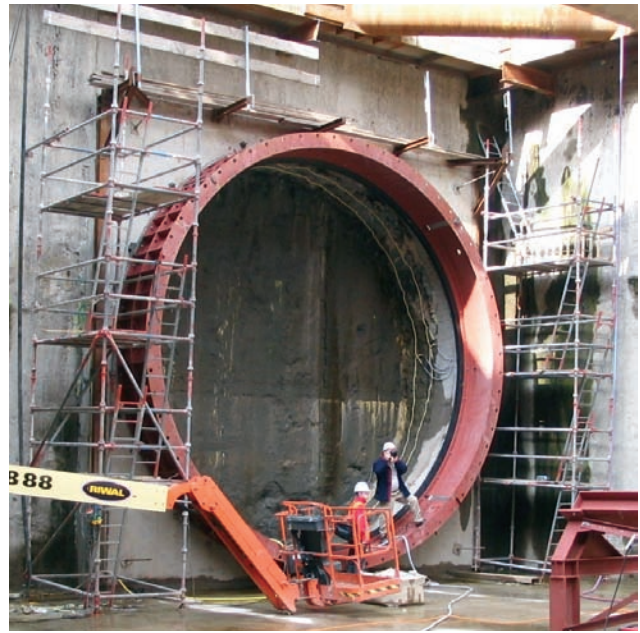
[Fig. 12] Sealing Construction
