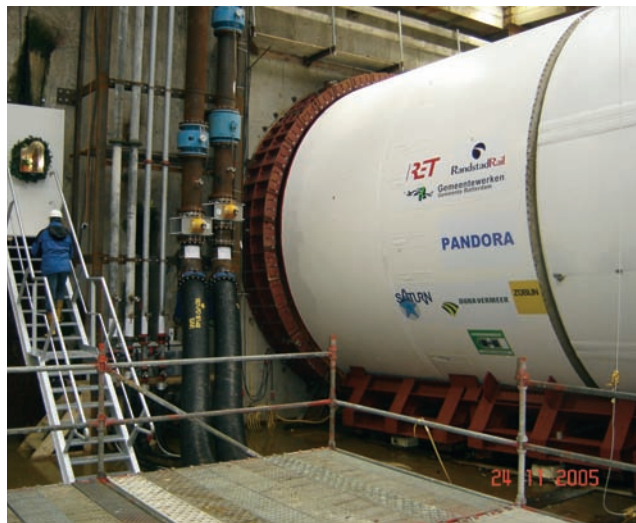
[Fig. 18] TBM in Start Shaft
