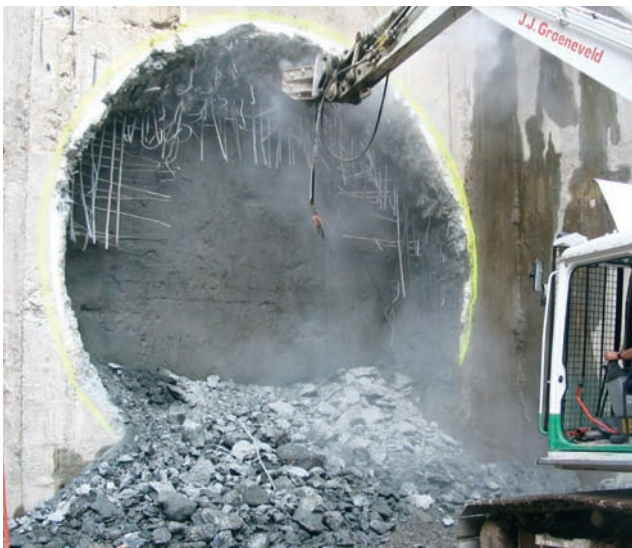
[Fig. 11] Opening of Diaphragm Wall
