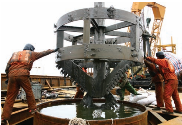
[Fig. 9] Drill Bit Exiting Hole
