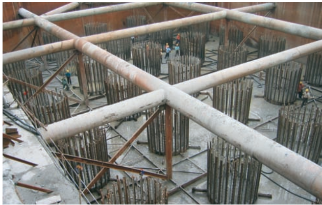
[Fig. 22] Dewatered Cofferdam and Top of Tremie Seal
