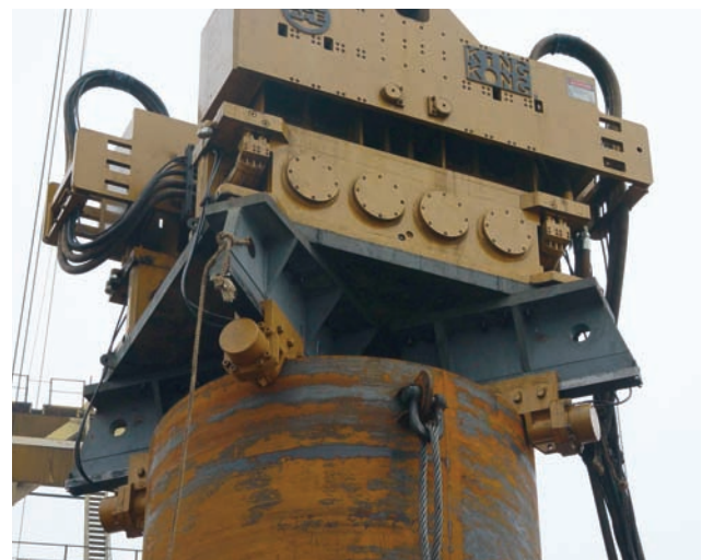
[Fig. 7] Casing Installation Hammer
