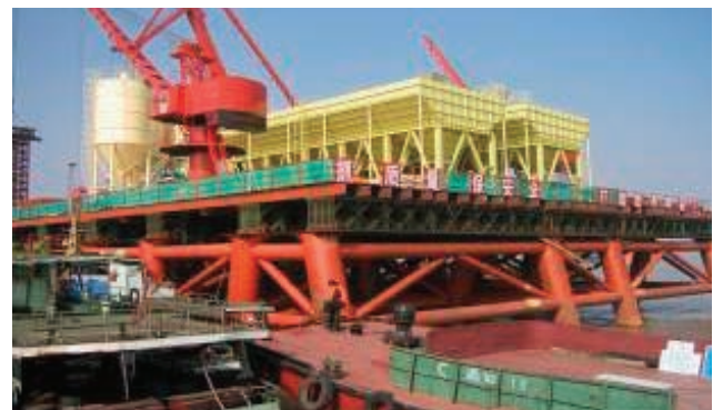
[Fig. 6] Batch Plant Platform
