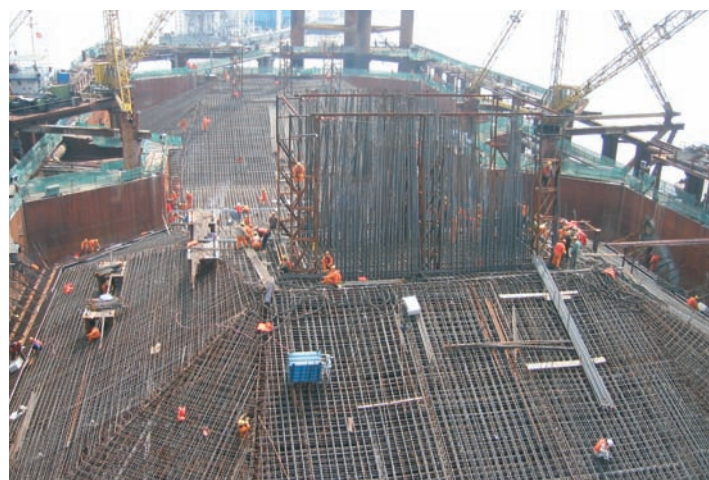
[Fig. 23] Completion of Pile Cap in the Dry at Pylon 4
