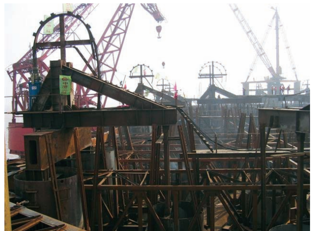
[Fig. 20] Strand Jack Model DL-S418 & Reaction Frames Inside Caisson at Pylon 4
