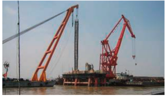
[Fig. 10] Reinforcing Cage Installation
