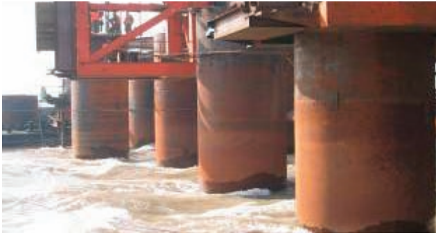
[Fig. 16] 3 m/sec Currents at Pylon
