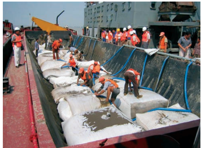
[Fig. 17] Filling Geotextile Bags
