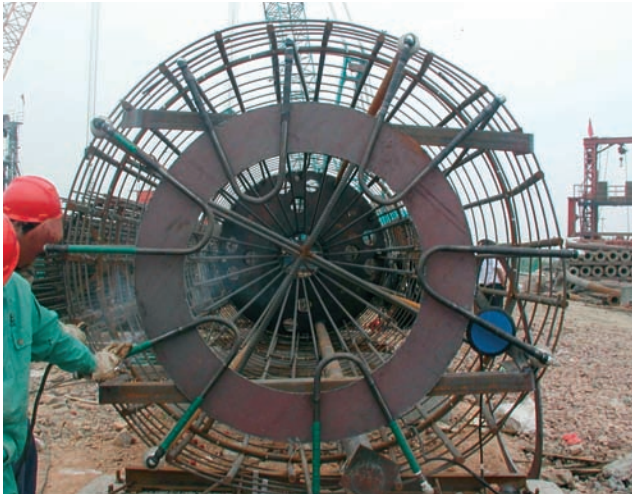
[Fig. 11] U-shaped Grouting Pipes at the Shaft Tip
