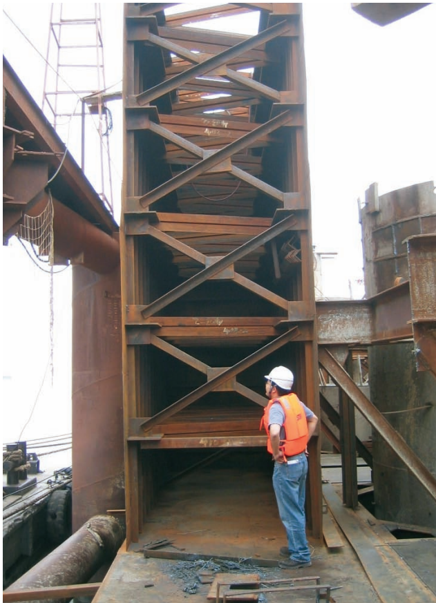
[Fig. 18] 2 m Thick Caisson Perimeter Wall
