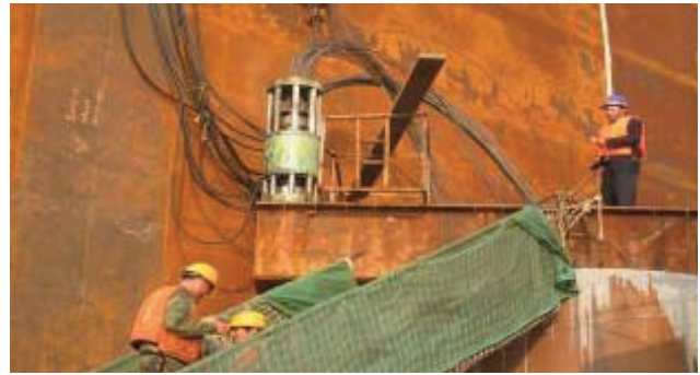
[Fig. 19] Typical Strand Jack at Pylon 5
