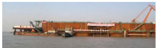
[Fig. 21] Pylon 5 Caisson Being Lowered
