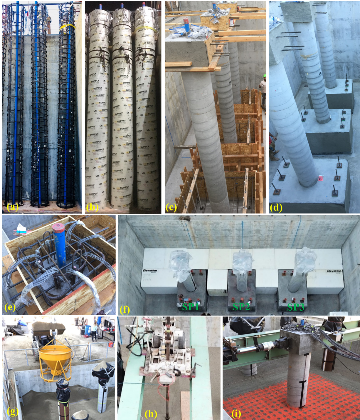
Figure 8. (a) Pile rebar cages, (b) Instrumented specimens prior to concrete pouring, (c) Concrete piles placed in rock-socket formwork, (d) Specimens with rock-sockets anchored into the floor (e) Pile cap prior to cap concrete pouring, (f) Geofoam blocks in place, (g) Sand pluviation, (h) Ramset setup for CPT/DMT testing, (i) Completed test setup for SP 1
